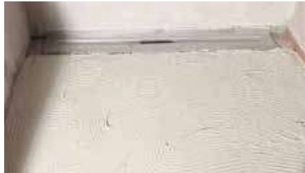
Apply a 1-2mm bed of tile adhesive evenly onto the floor.
