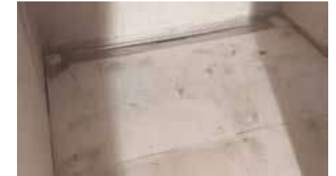
Place the UniSlope board and end fillers into position and screw down.
