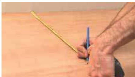
Mark and cut out the wet room area.
