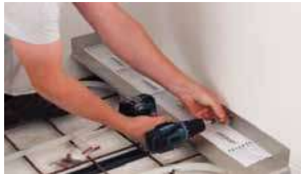
Screw drain to wall using screws supplied and connect pipework.
