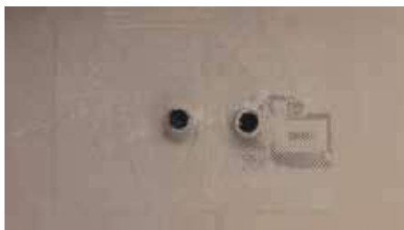
Reinforce around the first fix pipework ensuring there are no gaps.
