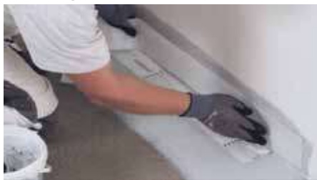
Apply VS30 using a brush or roller to all major joints. Place reinforcement tape into position.
