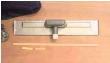
Attach push fit adapter into the outlet. Cut three battens to size.
