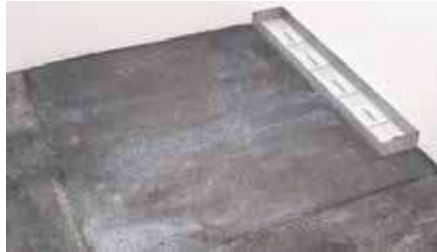
Allow approximately 30 minutes for Primer to dry. Ensure it is touch dry.
