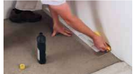
Degrease the drain using a degreasing agent.
