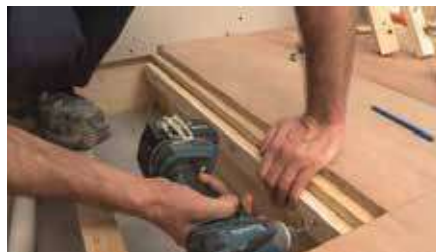
Install battens between the joists.
