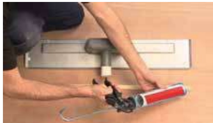
Apply glue to the battens.
