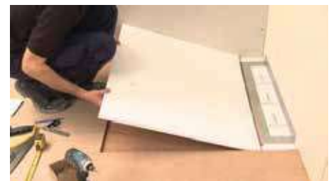
Screw the UniSlope board and end fillers into position using dry wall screws.
