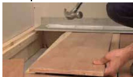
Cut the ply wood and place on top of the battens between the joists.
