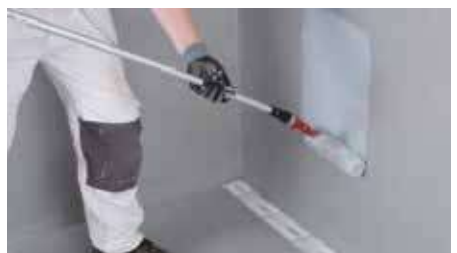
Allow to dry for 12 hours and ensure the first coat is touch dry. Once dry, apply second coat of VS30.
