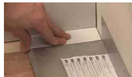
Place the UniSlope boards and end fillers into position.
