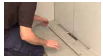
NO NEED TO CUT TILES TOWARDS DRAIN
