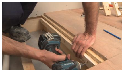
Install batons between the joist.
