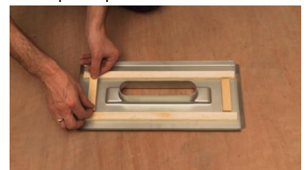
Place onto the bottom of the main drain body.
