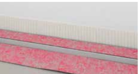
Using adhesive, apply membrane to floor & wall. Smooth to remove bumps.
