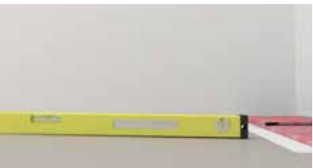
Slope the floor 1.25% to 2% to the drain.
