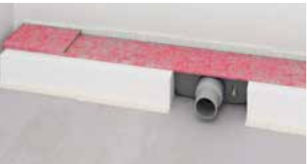
If using the polystyrene support, bed into adhesive.
