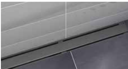
Place the Tile Insert / Panel / Tiled base into position.
