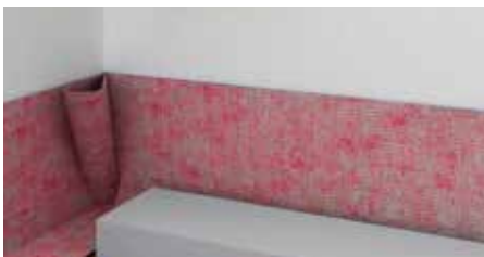
Cut the corner where the membrane overlaps.
