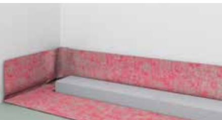
Place fitted membrane into position.
