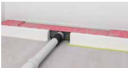
Connect pipework to the drain allowing for slope in pipe.
