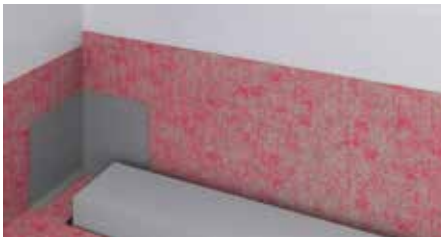
Stick plastic corner pieces onto the glue.
