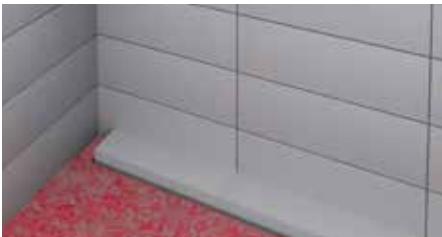
Waterproof remaining areas and tile the walls and floor.
